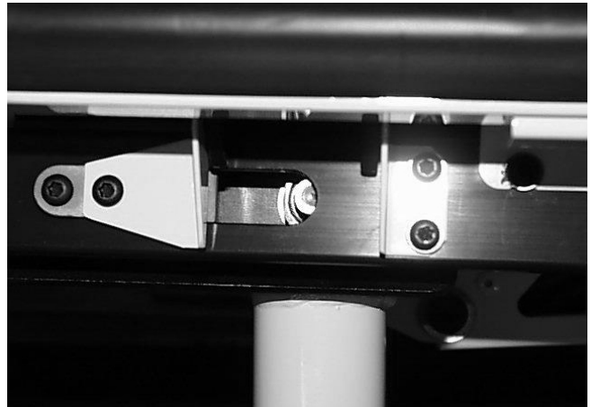
Figure 36 – Locking Pin Not Properly Engaged
