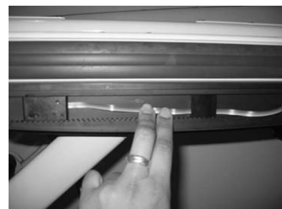
Figure 4e - Securing Cables
