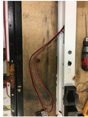
Figure 7 – Run the wire alongside the anchor
