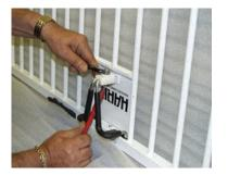
1. Turn rail upside down and remove acorn nut and lock washer from the retainer block.
