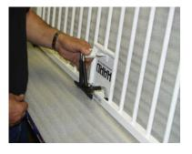
9. The trigger barrels are spring loaded, so to line up the hole in the trigger barrel with the hole in the bracket and opening in the rail, push in on the white plastic bushing on the end of the trigger until the holes line up on one side, then insert one half of the handle. Repeat on the other side and insert the second half of the handle.
