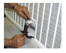
10. To insert screw in the retaining block through the metal bracket in the shield plate, twist the retaining block and screw up into the hole from an angle and secure with lock washer and acorn nut.
