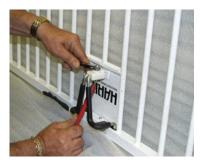
1. Turn rail upside down and remove acorn nut and lock washer from the retainer block.
