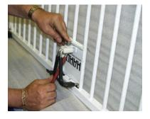
10. To insert screw in the retaining block through the metal bracket in the shield plate, twist the retaining block and screw up into the hole from an angle and secure with lock washer and acorn nut.
