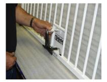
9. The trigger barrels are spring loaded, so to line up the hole in the trigger barrel with the hole in the bracket and opening in the rail, push in on the white plastic bushing on the end of the trigger until the holes line up on one side, then insert one half of the handle. Repeat on the other side and insert the second half of the handle.
