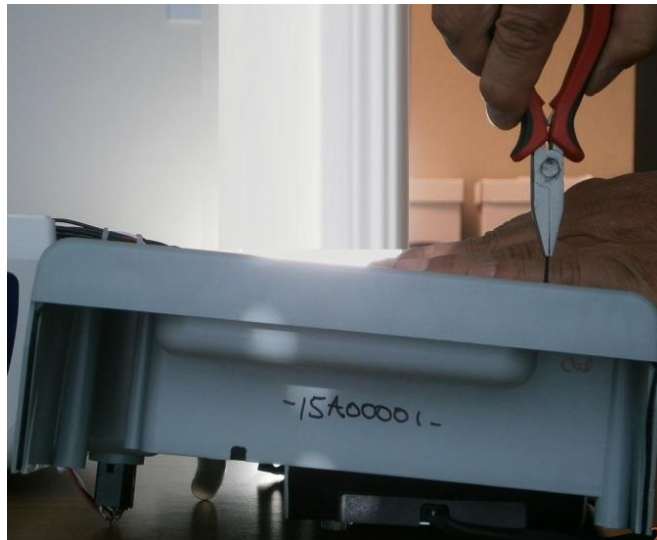
Figure 32: Locking anti-vibration mounts on the back case
