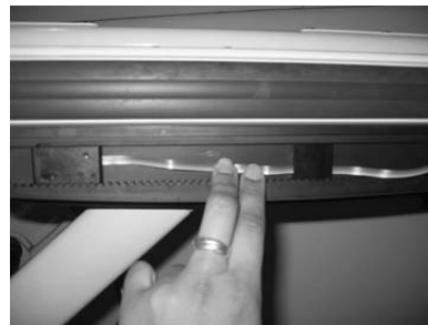
Figure 4d - Securing the Cables
