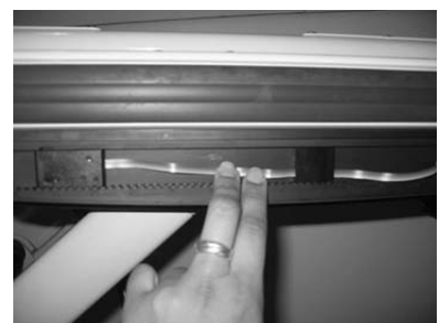
Figure 4e - Securing Cables
