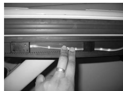
Figure 4e - Securing Cables
