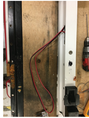
Figure 6 – Run the wire alongside the anchor
