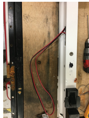
Figure 7 – Run the wire alongside the anchor
