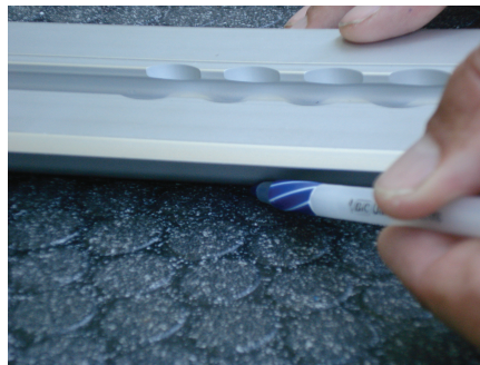
Figure 1 – Trace the floor plate
